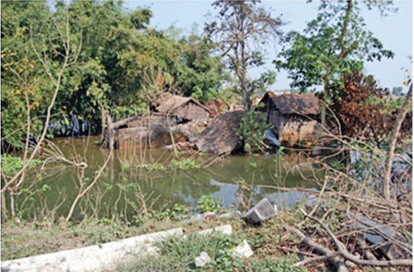
2008 Flood: Devastated rural homes in lower Koshi
