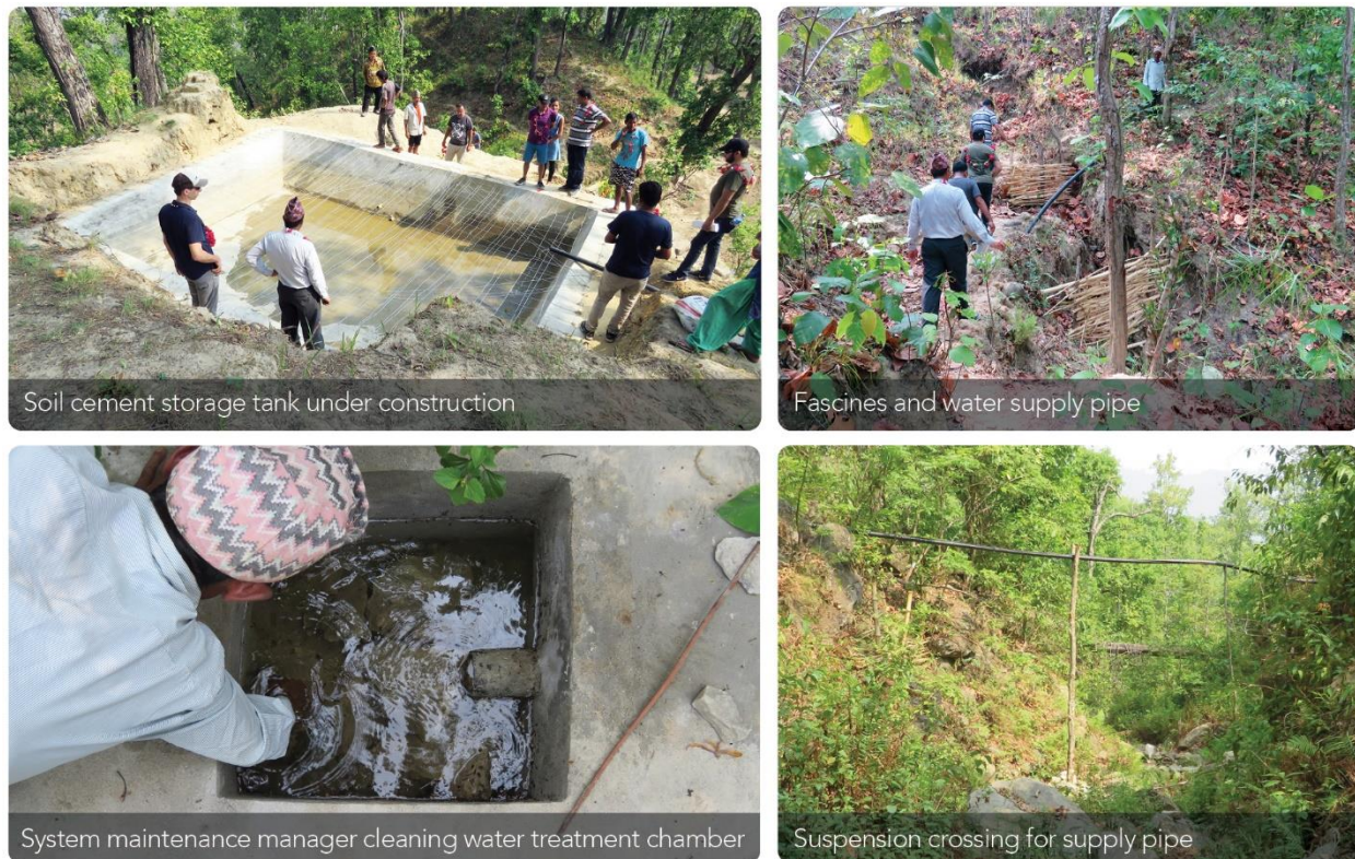
Figure 6: Milan Debari irrigation infrastructure and bioengineering constructed by PAHAL
