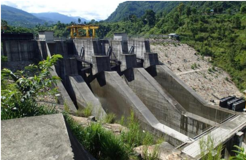
Figure II-3: Current dam design with either limited or no provisions for upstream of downstream aquatic species. (M. Weinhold)
